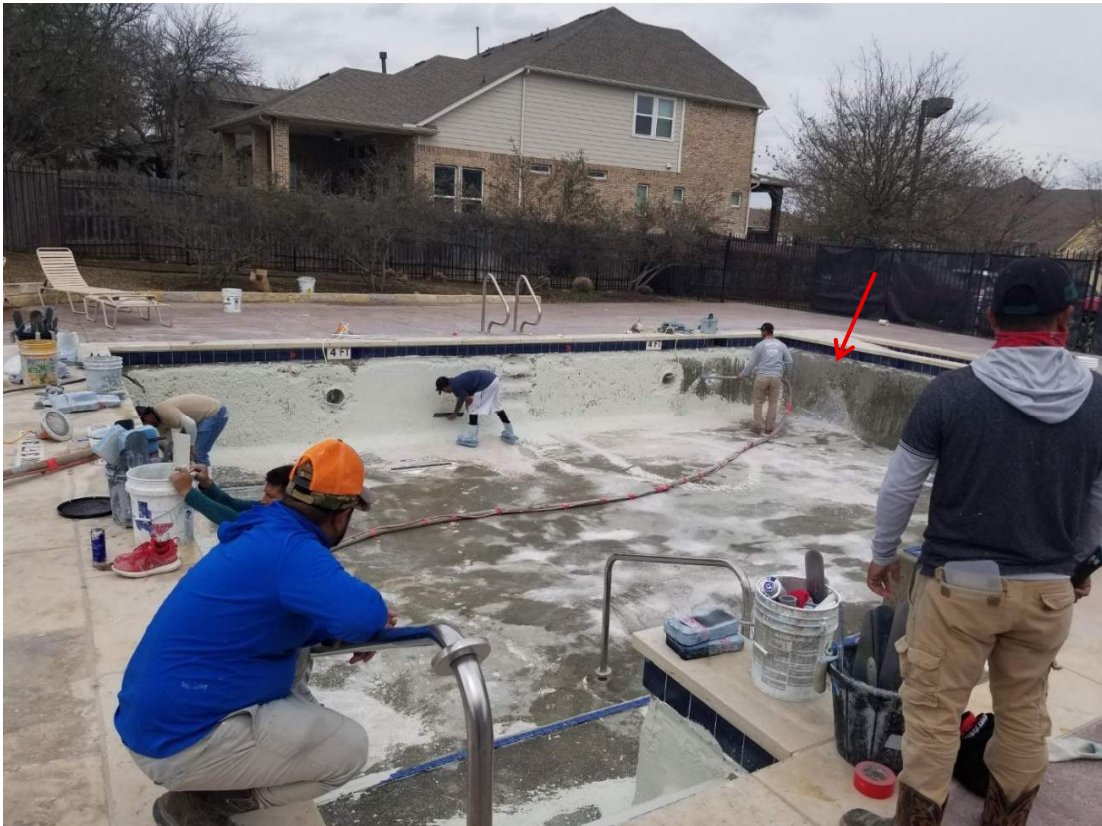
Photo No. 2 (2021) - New plaster applied over the bond coat.
